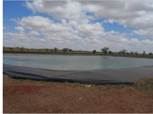
Constructed dam for drip irrigation in Chinangali 2
