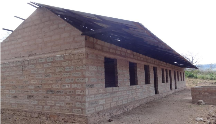
Image 22. Two new primary school classrooms at Uleka sub-village.
