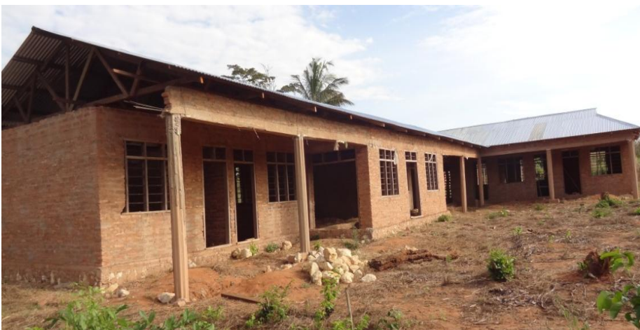
Image 23. Dispensary building under construction in Nandambi Village.
