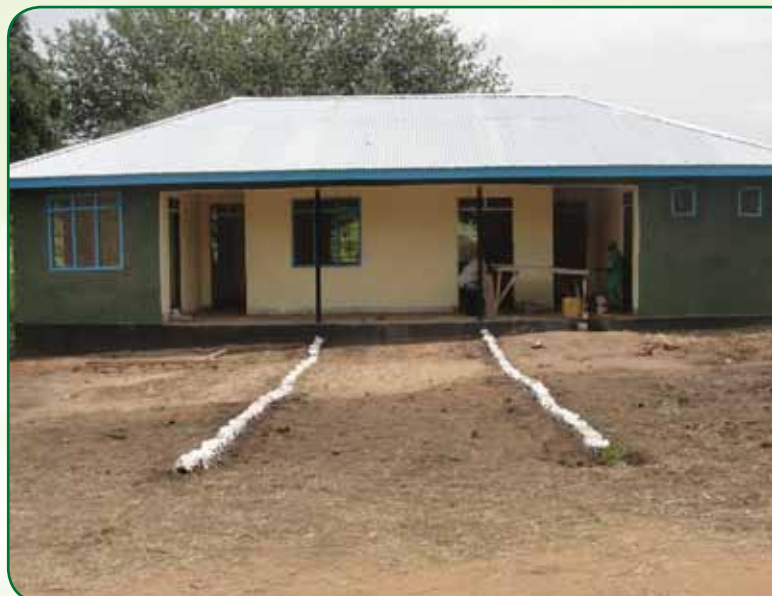
The Chabima Village Office, constructed with support from the project.
