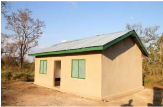
Construction of medical officer house at Ihombwe Village
