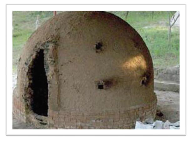
Figure 21: Half Orange Brick Kiln<sup>56</sup>
